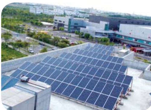
Solar panels installed on the roof of the Tainan factory.
